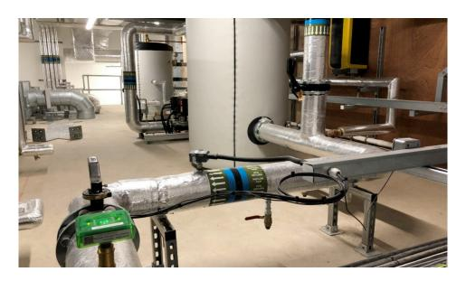
The carbon steel used on this project is 1.2mm (1200µm) thick and the initial fill passivation we noted earlier, on a well-designed system may average around 0.005mm (5µm) per year. This may not remain constant (uniform corrosion) depending upon numerous factors but suffice it to say if AYCR isn't measured, then it will never be possible to improve outcomes.
