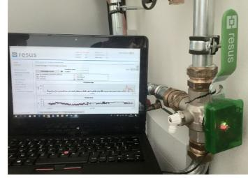
These alarms give operators and FM companies plenty of time to check, locate and remedy the causes of the increased corrosion levels before they do any costly damage to the system. This goes even for systems with thin wall carbon steel pipework for which corrosion monitoring is a must for routine maintenance and correcting simpler problems a smart system could definitely have its advantages'.
